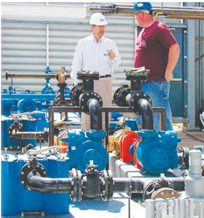
Shown in photo above: Blackmer Pump, HXL-12, 100 HP, 2200 GPM
